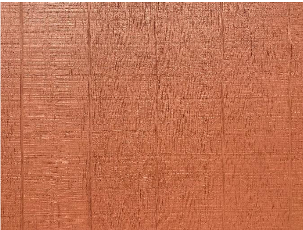
Plate 15: Vertical Plank Siding
