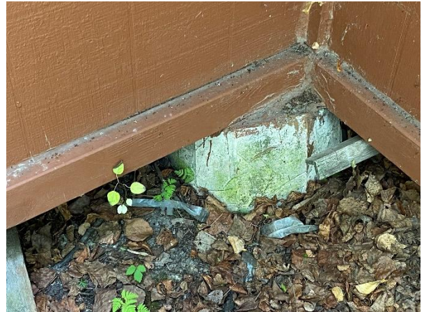
Plate 14: Concrete Foundational Support
