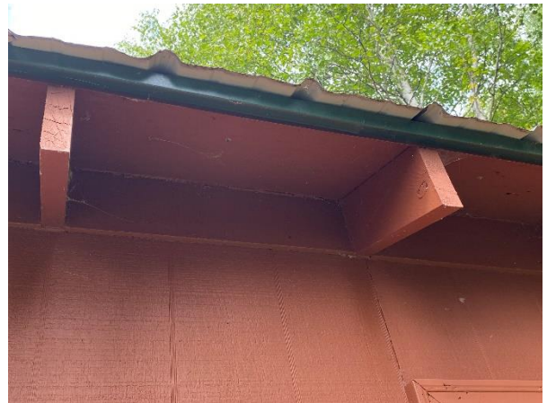
Plate 16: Projecting Eaves with Exposed Rafters
