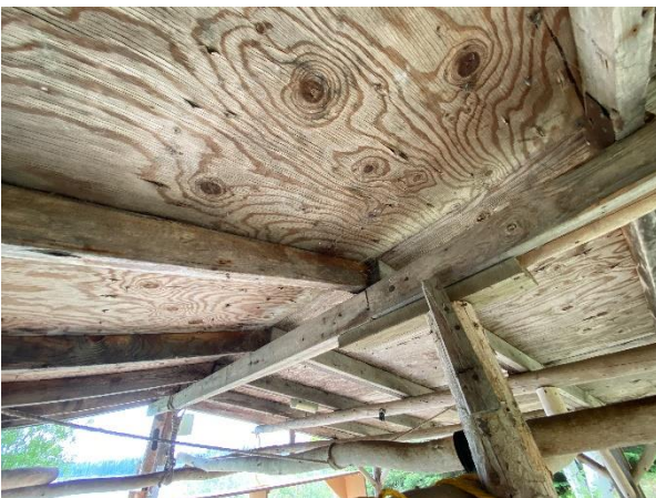
Plate 21: Roof Supports of Sheltered Gazebo Work Area
